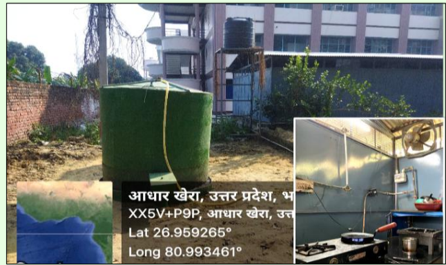
Biogas Plant of 20 m 3 Capacity
